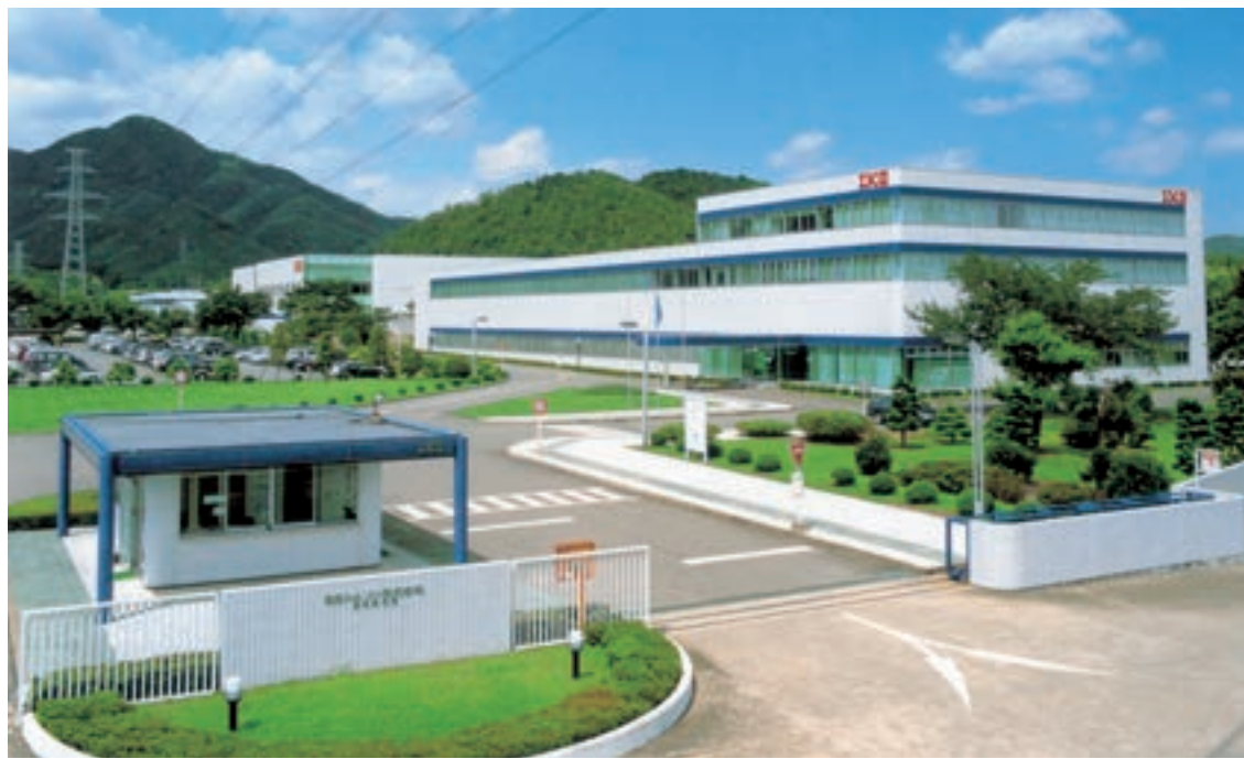
Main entrance of Gifu plant
